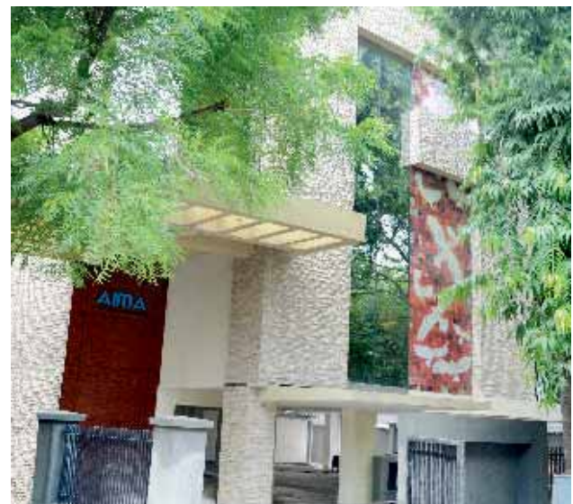
AIMA's new Office Building
