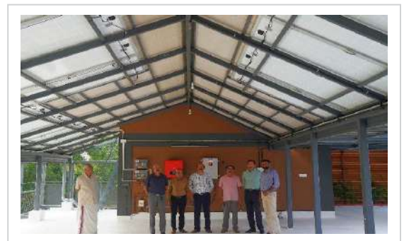
Team under the integrated solar roofing system
